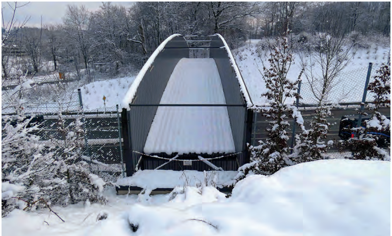
Figure 13: Crossing aid for bats (ATP GmbH)
